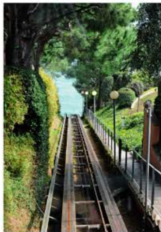
Funiculaire conduisant au studio Renzo Piano. The funicular leading to Renzo Piano's studio.
